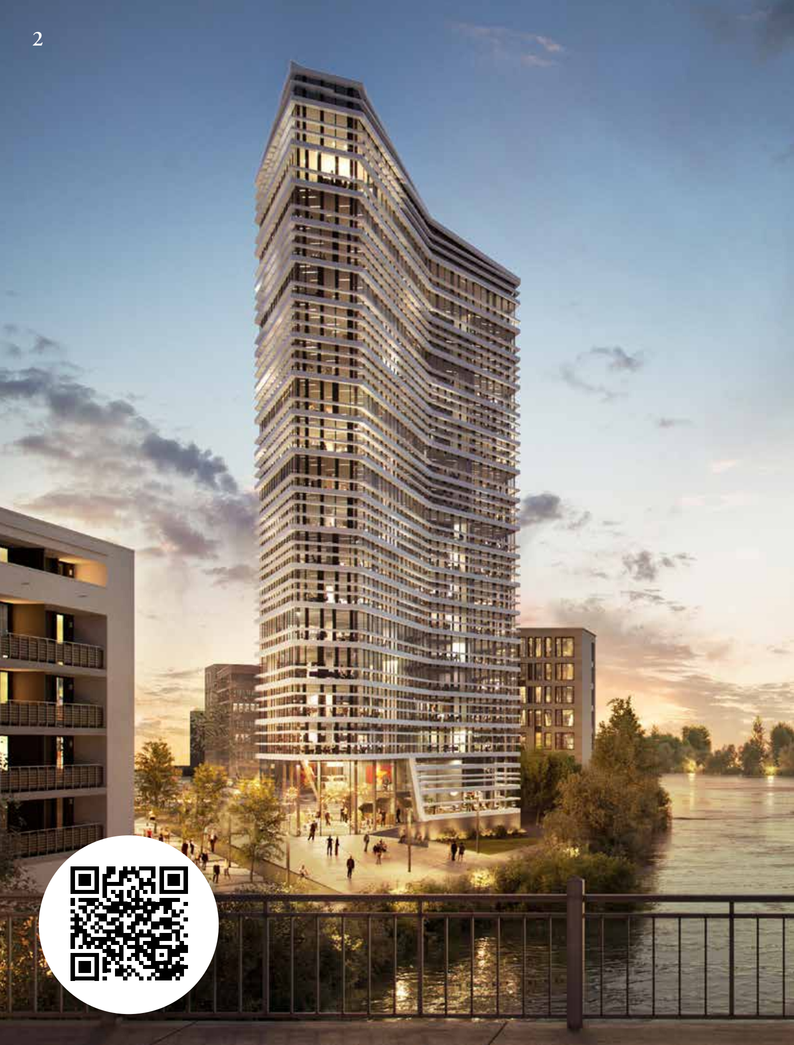
WAYV Riverside Office Tower, Offenbach, Deutschland
